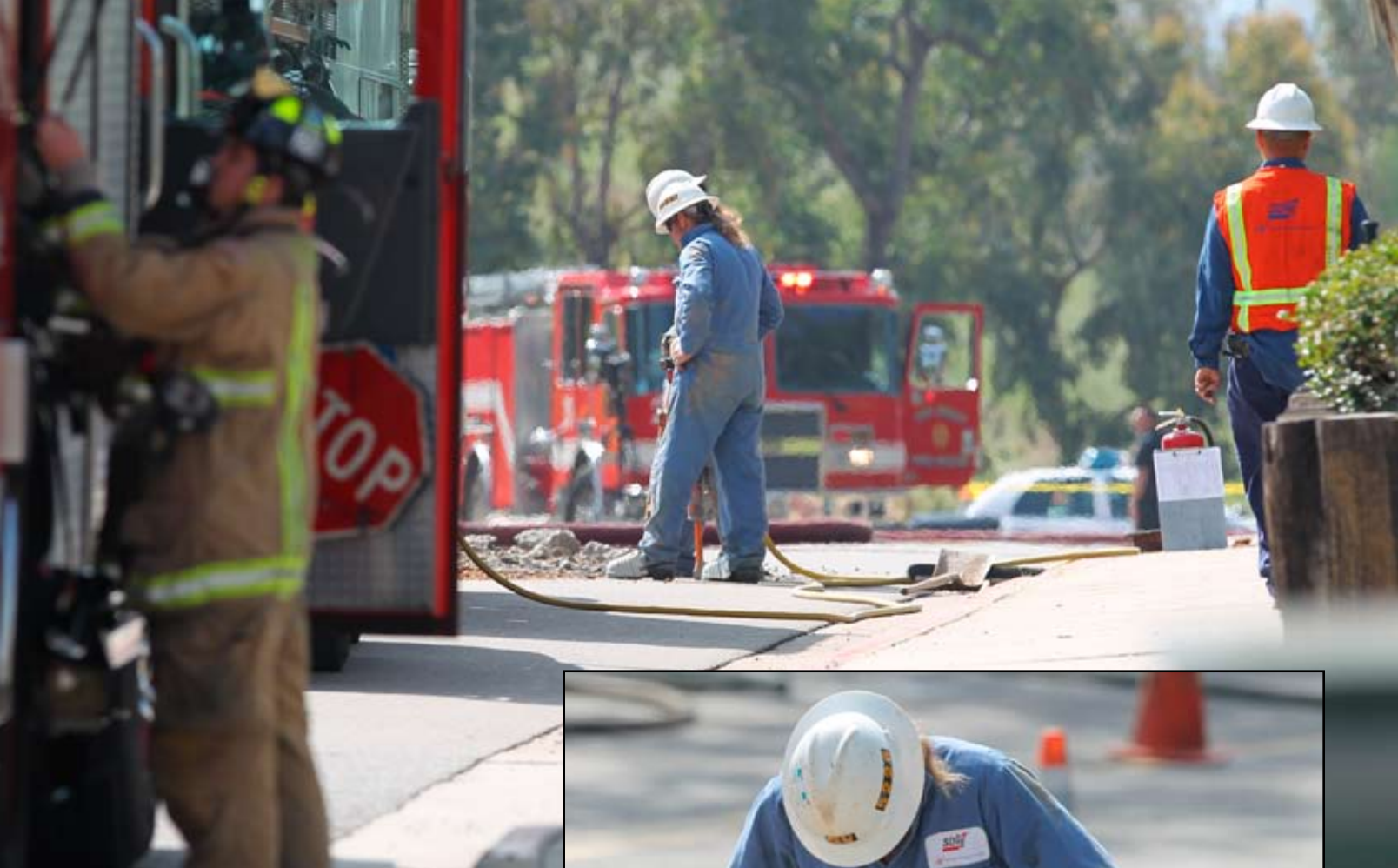
Gas company workers break pavement on the opposite side of the street from the leaking gas. Here, the gas service will be crimped in order to stop the flow of gas.
