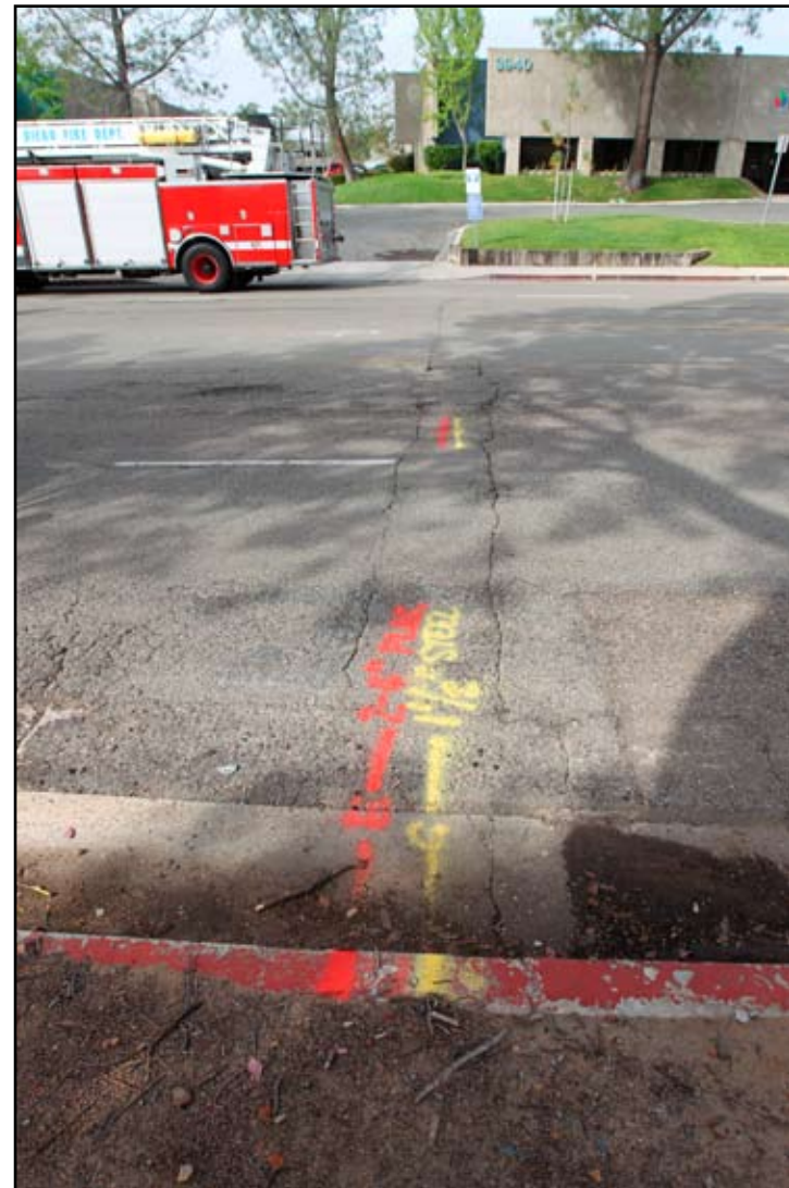
Pavement cracks are visible at this marked gas and electric joint trench located just outside the safe zone. The utility workers were trenching in this direction when they struck the unmarked gas service.
