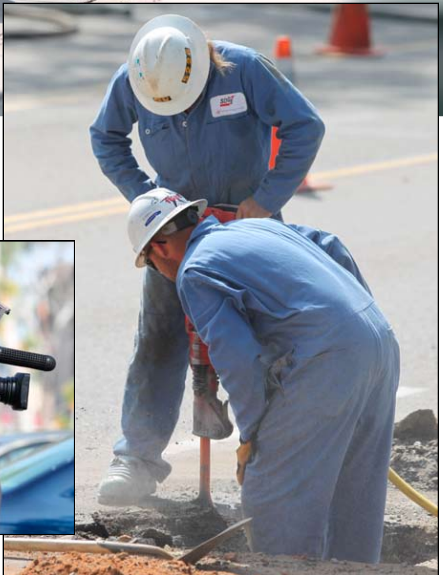
Gas company workers break pavement on the opposite side of the street from the leaking gas. Here, the gas service will be crimped in order to stop the flow of gas.
